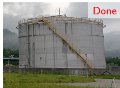
5000 m 3 LAB tank
