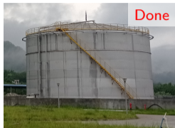
5000 m 3 LAB tank
