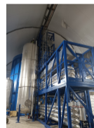
Gas stripping: remove Rn and O 2
