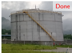
5000 m 3 LAB tank
